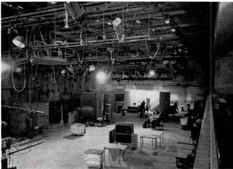
FIG. 28, ABOVE: LIGHTING ARRANGEMENT EMPLOYED BY WHAS-TV. FIG. 29, BELOW: COUNTERWEIGHTED BATTENS SUPPORT FIXTURES IN WNBT STUDIO 8H
