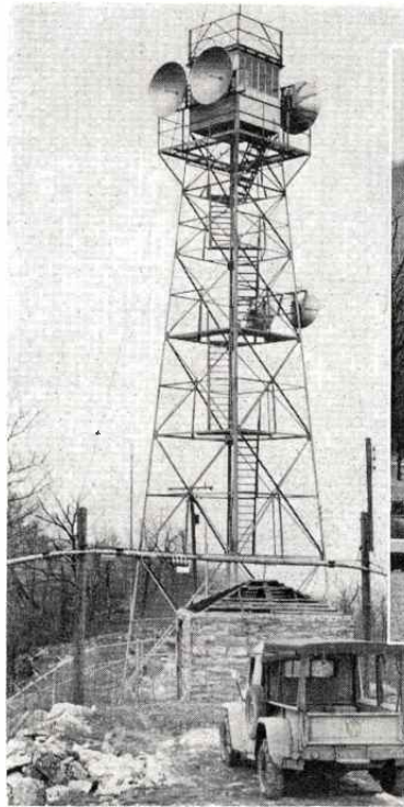
LEFT: UHF RELAY AT TUSSEY HAS LINK TO EVERETT BUILDING. AT & T TRANSCONTINENTAL CABLE CROSSES MOUNTAIN AT THIS POINT. BELOW: LINE-OF-SIGHT TO TUSSEY RELAY
