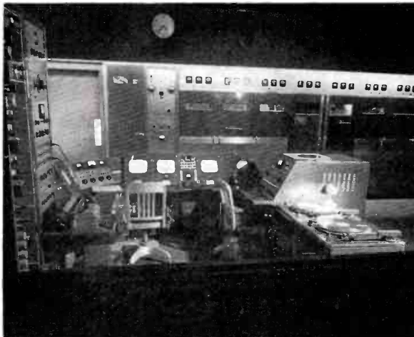
FIGS. 14, 15. MASTER-CONTROL AREA OF KRON-TV IS U-SHAPED FOR MAXIMUM OPERATING CONVENIENCE. DIRECTOR FOR LIVE SHOW STANDS IN THE U
