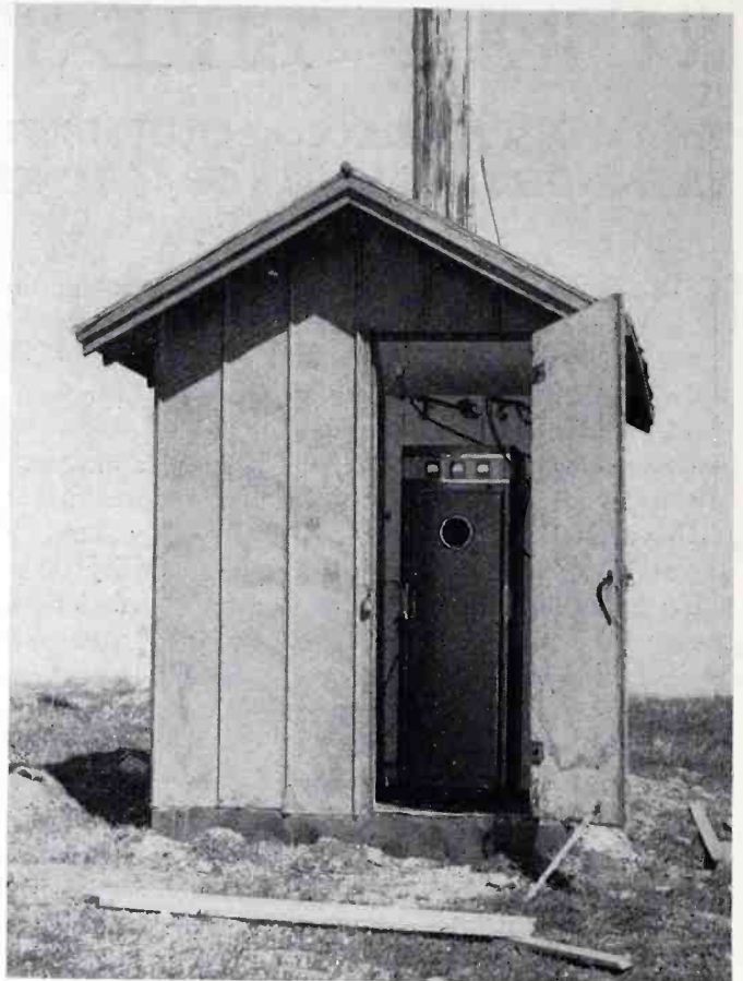
FIG. 2. PARIS HILL REPEATER STATION. NOTE ANTENNA SEPARATION. FIG. 3. HOUSE FOR REPEATER RADIO EQUIPMENT AND STANDBY GENERATOR
