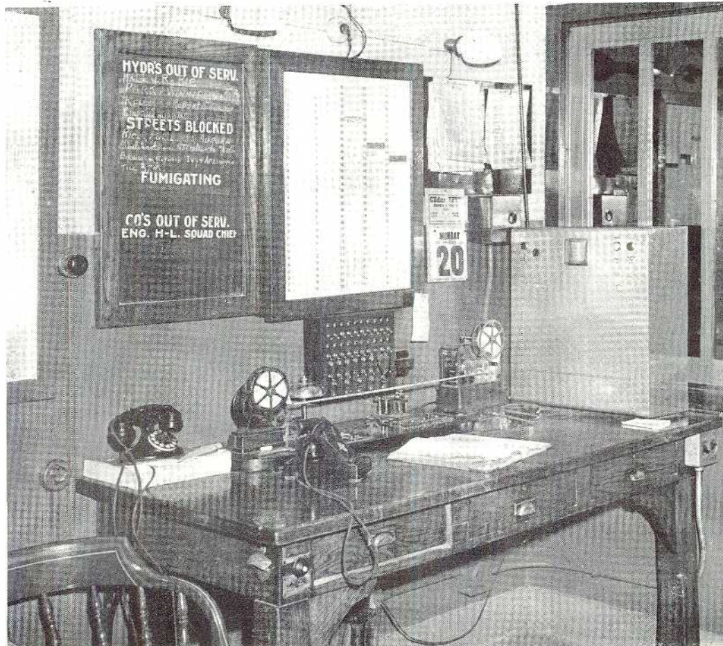
FIG. 5. AT THE RIGHT IS A SELECTIVE-CALLING RECEIVER INSTALLED AT ONE OF THE FIRE HOUSES
