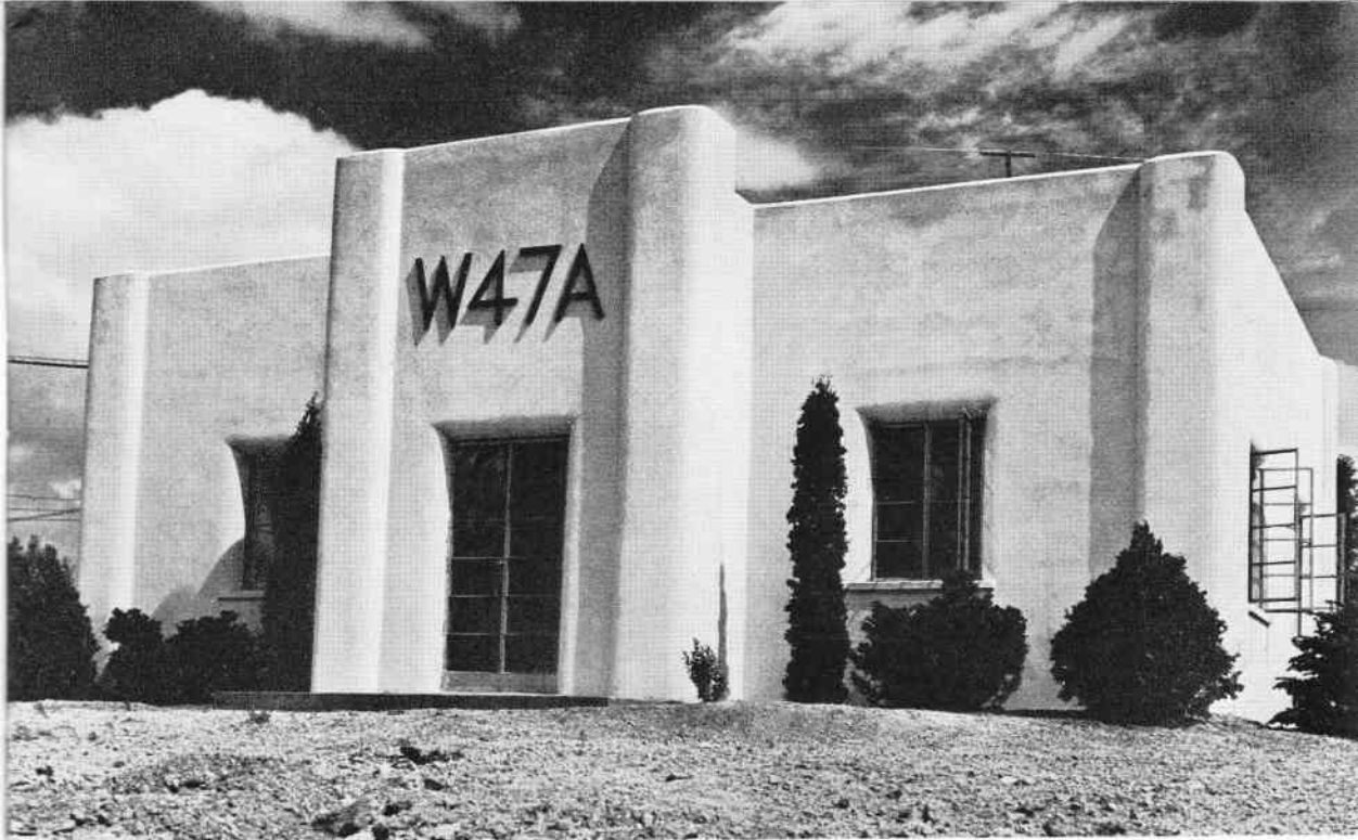
W47A TRANSMITTER HOUSE TOPS MT. PINNACLE, 1,600 FT. HIGH, NEAR ALBANY, N. Y.
