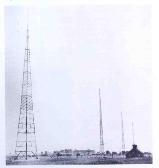
Fig. 2. Array at WCAO, with new No. 1 tower and FM antenna in the foreground
