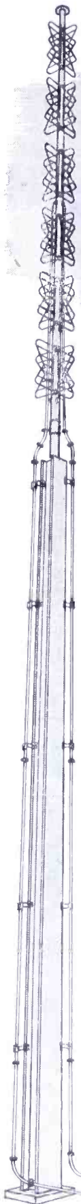
Television antenna of WGN-TV — Chicago's newest and most powerful television station—showing Andrew 1-5/8" flanged television transmission line.
