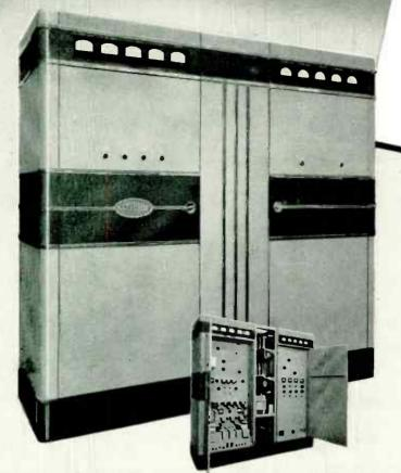
Front view shows arrangement of controls for tuning driver and amplifier, Center lift-off panel has been removed to show accessibility of power supply.
