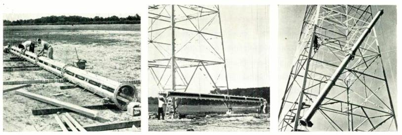
Assembling the sections into one unit
