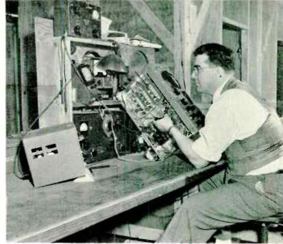
11: CIRCUIT CONTINUITY IS CHECKED AT END OF THE LINE. 12: OSCILLATOR ADJUSTMENT IS LAST STEP BEFORE TEST CAGES
