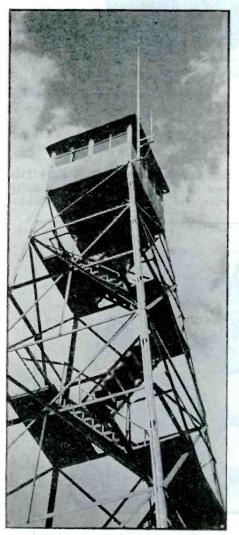
FIG. 4. ADJUSTABLE COAXIAL ANTENNA OF THE TYPE USED FOR 70 MC.
