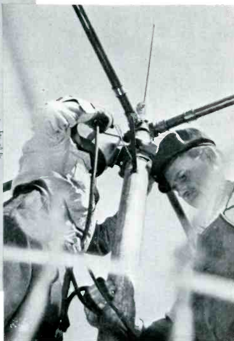
LEFT, W45D USES DE MARS TYPE OF 2-BAY TURNSTILE, 700 FT. ABOVE THE STREET LEVEL
