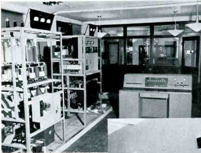
ABOVE, RECTIFIER AND CONTROL UNITS IMMEDIATELY AFTER DELIVERY.—RIGHT, SIX WEEKS LATER THEY WERE COMPLETELY INSTALLED, TESTED, AND READY FOR SERVICE
