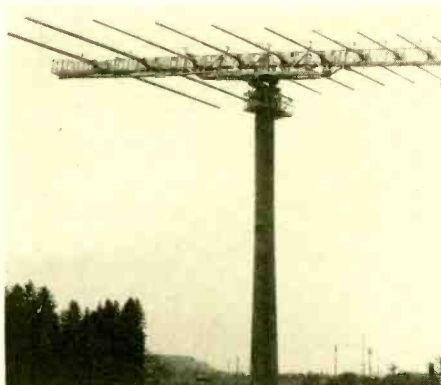
Here's the log-periodic antenna used for the 250 kw transmitter at Schwarzenburg.
