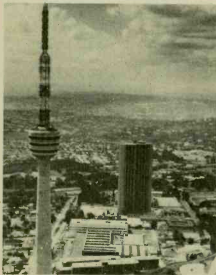
This is the 40-acre site of the Broadcasting Center in Johannesburg, home of RSA as well as television and FM radio stations.
