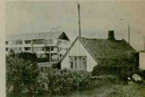
This old house in Reykjavik, Iceland was made of turf and stone around a wooden frame the way houses there were until recently.
