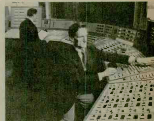
This shot of the Bush House Control Room operating desk will give you an idea of the vast complexity needed to run the BBC system.
