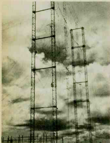
Trans World Radio's massive antennas beam 500 kilowatts medium wave and 250 kilowatts shortwave from the Bonaire, Netherlands Antillies station. This station also relays transmissions for Radio Nederland.
