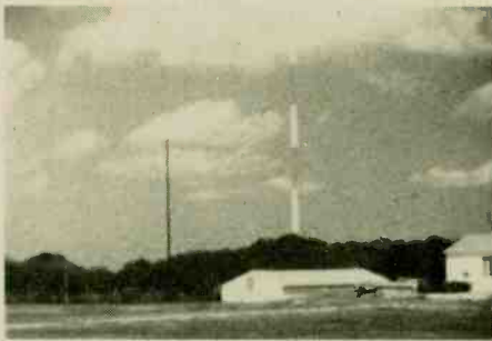
One of the transmitter buildings is seen here near the base of a 250-ft. antenna tower. Two 50-kilowatt transmitters supplied the output power for Radio Swan.
