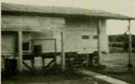
Mobile equipment trailer was built in for a long stay. Note concrete path and roof supported over trailer.
