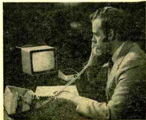
The Videovoice system transmits still black-and-white TV pictures over the same circuit used for a voice conversation. The photo above illustrates how a diagram under discussion could be transmitted. The photo below demonstrates the receiver end.
