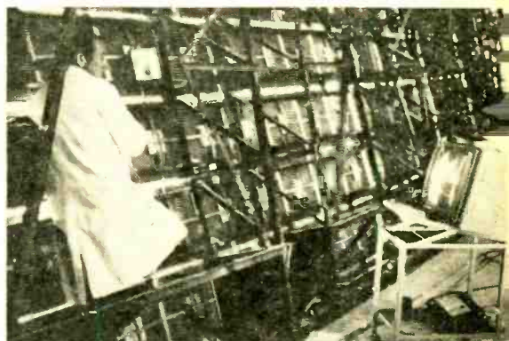
Many mirrors located inside complex demand individual attention to focus them on central focal point inside laboratory's oven. Here, one of Odeillo's engineers relies on TV hookup to aid him in zeroing in on sun.
