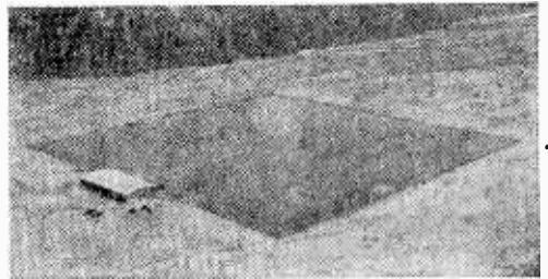
Fig. 10. Broadside antenna covers 25 acres near Lima, Peru. This radar probe uses a 6-megawatt transmitter.
