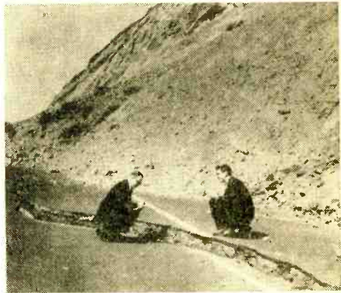
Because San Francisco lies in a major earthquake belt, 1906 could repeat itself at any time. Above, 1957 fissure on coast road just south of the city.
