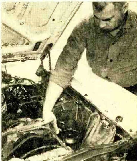
Trumpet speaker mounts under hood in forward position. But toggle switch under dash will cut it out fast so passersby won't worry about your talking engine!
