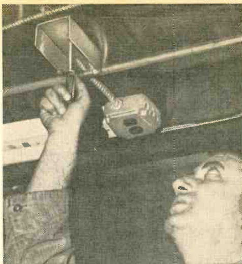
Install bottom of base box in convenient location close to bell wires and AC outlet. Attach transmitter half of box; then just set it and forget it—you'll always hear the bell.
