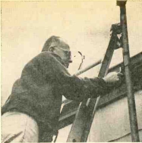
It's easy to install the base antenna 2 by using standard TV antenna hardware. The mast can be attached to the side of the house using mast clamps.
