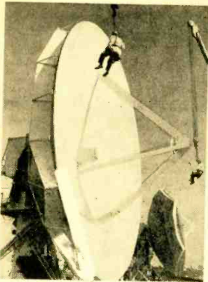
Technicians, dangling in bosun chairs (left), are dwarfed by 40-foot diameter parabolic antenna. Air-transportable terminal is set up in 48 hours.
