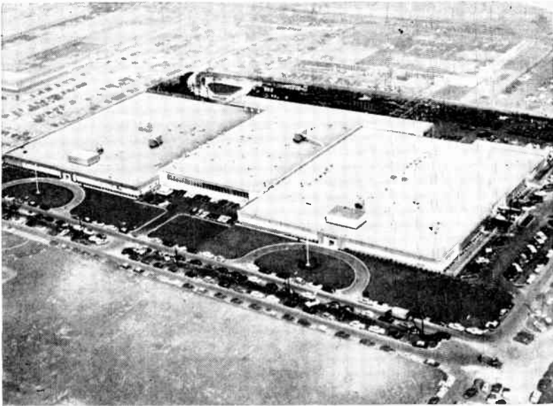
REEVES' new Mincola plant shows how Long Island provides . . .
