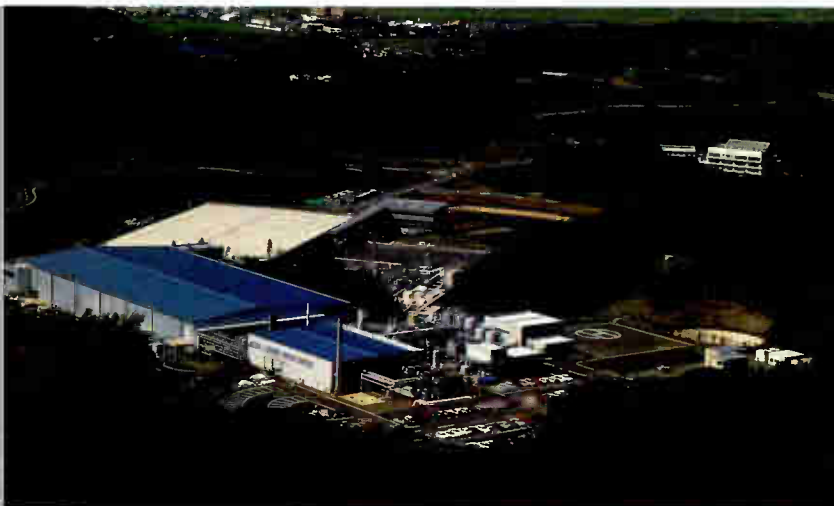
Our three manufacturing plants: Modules I, II, and III
