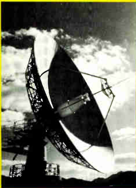
Cassegrain 13-meter diameter antenna at MARISAT shore station in Yamaguchi, Japan.
