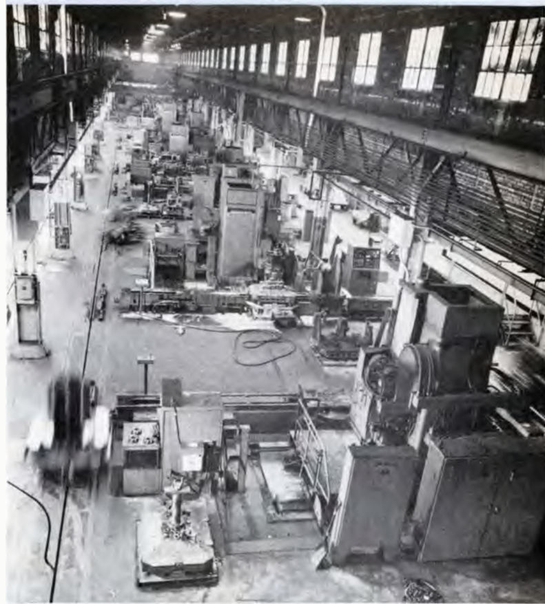
6. Automated shop. Tow carts (blurred by motion) deliver castings at the Allis-Chalmers plant to the appropriate tool. Castings are automatically loaded onto the tool, machined, and unloaded.
