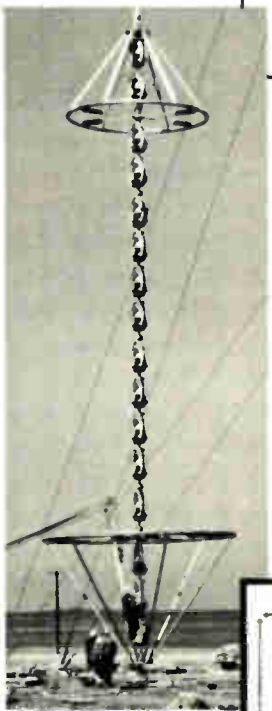
Large structural-guy insulator assembly with grading rings
