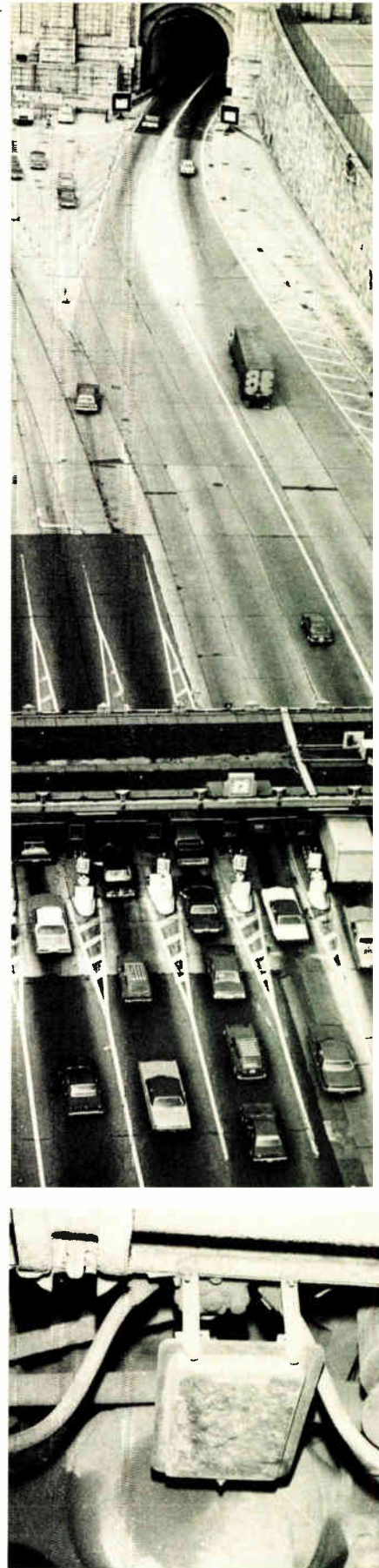
Taking tolls. Lincoln Tunnel toll booths would be a memory if automatic vehicle identification becomes universal. Transponder is shown mounted beneath bus.
