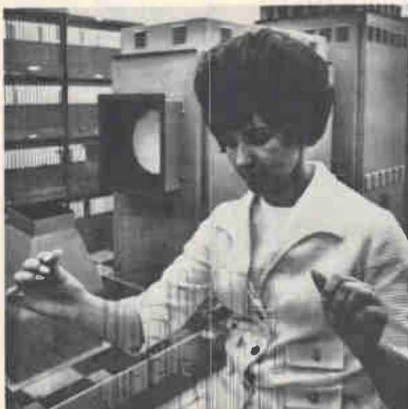
Representational art. Univac's new display unit produces multi-layer-board artwork with a tolerance of \pm 2 mils in 15 inches.
