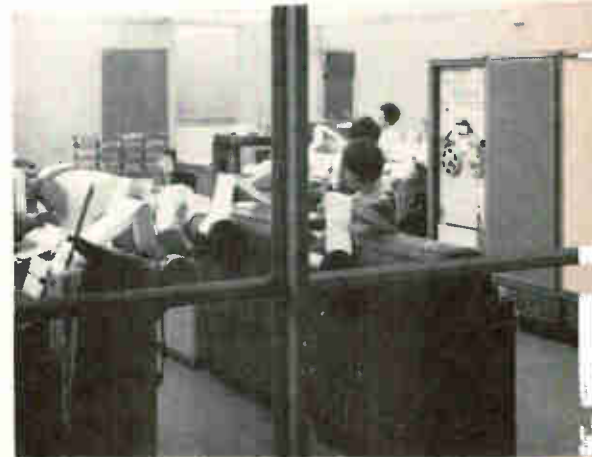
Keeping track. Switching system, right, controls traffic on multicircuit teletypewriter network.
