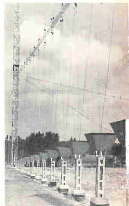
Weighted antenna. Lower ends of rhombic dipole elements in West German antenna are held down by weights that can move up and down.
