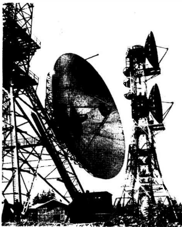
German Federal Post Office will have 100-mile Telefunken-built microwave link between West Germany and West Berlin in full operation by mid-1967. But cutback in Post Office budget for communications will depress microwave market next year.
