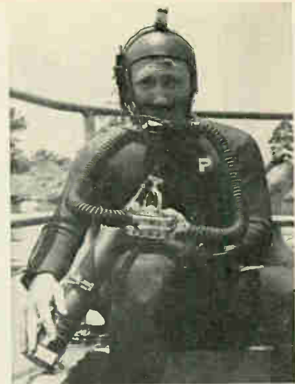
Aquasonics communicator is a 42-Kc a-m, device with 1,000 foot range
