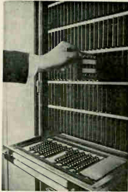
Mail sorting is masterminded from central electronic rack at left, which provides memory and logic. Girl at right stamps zip-code destinations on envelopes, which are sorted in the chandelier-like tower to her right.
