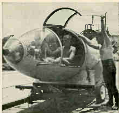
Wet submarines travel at 9 knots but are too maneuverable to use at deep levels where a quick ascent would be dangerous to aquanauts. The miniature sub might be used by surface divers to take supplies to Sealab.
