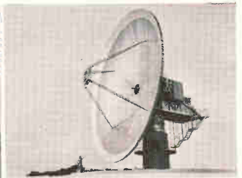
■ 20 meter diameter antenna for satellite communication
