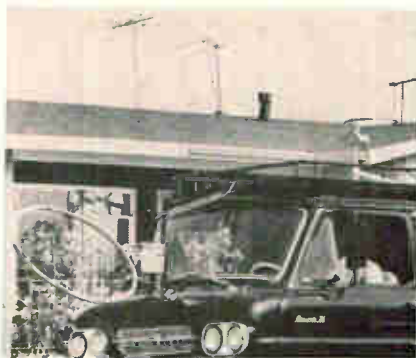
Truck cruises along residential street, picking up tv signals and recording the viewing choices of the residents.
