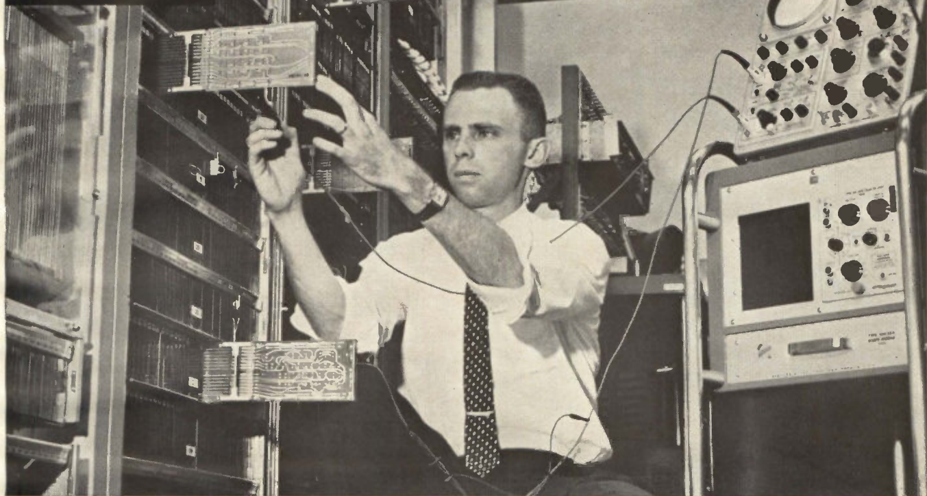
Bell Laboratories' E. G. Hughes tests printed circuit boards in experimental central office control equipment for 101-Electronic Switching System. The system automatically detects trouble, switching out a defective unit and switching in a duplicate unit so service is not interrupted.
