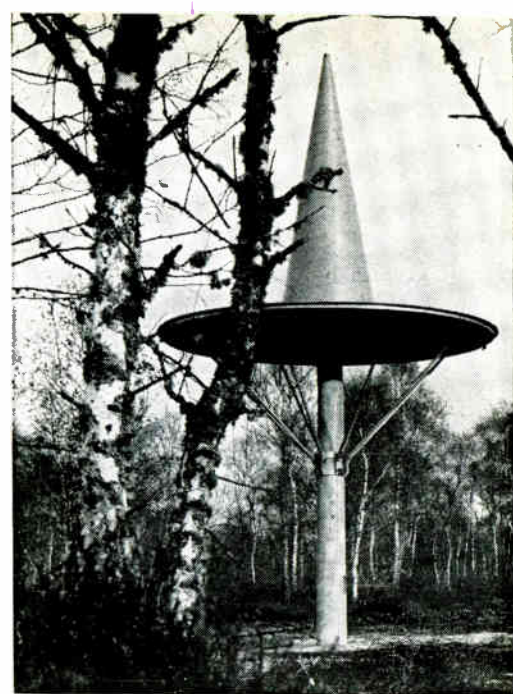
HELICAL ANTENNAS for experimental CSF width, give accuracy of 100 microradians
