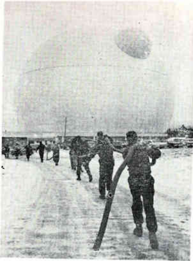
Antennas at main ground station at Andover were erected this winter under a huge inflated dome
