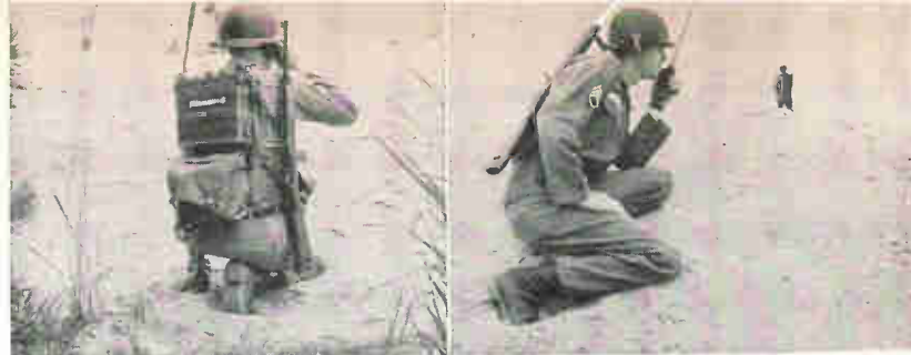
MICROMODULES will be used in a family of combat radios. At left is the conventional AN/PRC-25 case now equipped with micromodule circuits. At right is the AN/PRC-51 micromodule radio transmitting, with micromodule receiver clipped to the soldier's helmet
