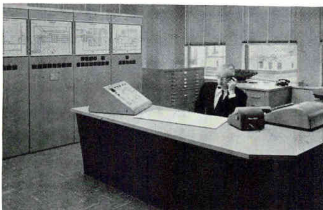
Automatic data acquisition and display gives true "fingertip" control to dispatcher J. H. Philips, enabling him to distribute peak day-loads up to 750 million cubic feet of gas to Peoples' 275,000 customers.
