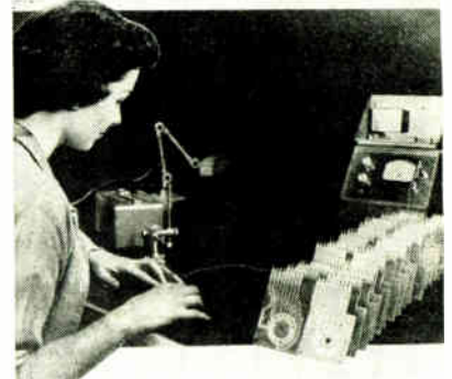
Conductivity tests for gold plated printed circuits
