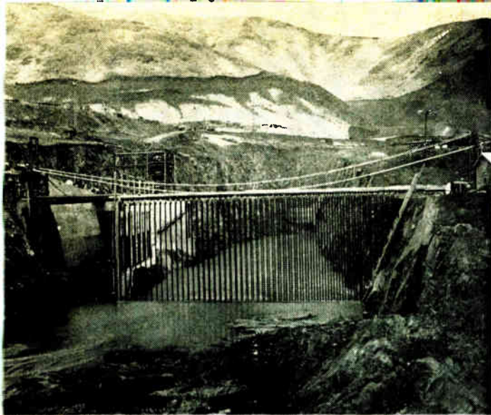
Electric fence (left) under construction at Brownlee dam site. Fish traps are seen through opening on left. Fence in use (right) prevents fish fighting upstream against current in diversionary tunnel, directional electric field urges them into fish traps where they are caught and transported past the diversion
