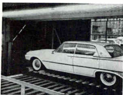
Car is lifted from parking station by fingers of elevator
