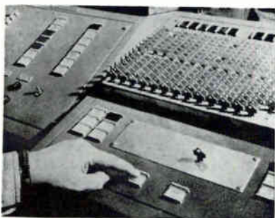
Key inserted in control board selects parking stall
