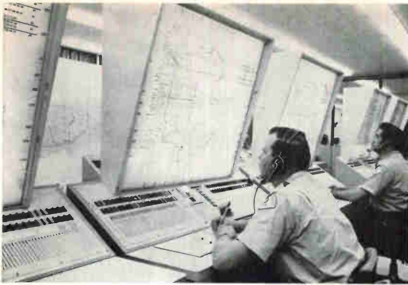
Consoles include patrol zone maps. Lights on map indicate availability of each of 80 patrol cars in the zone
