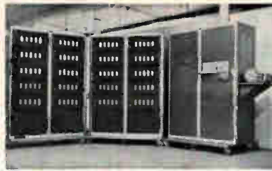
Automatic continuity tester checks wire-wrap assemblies for Polaris
