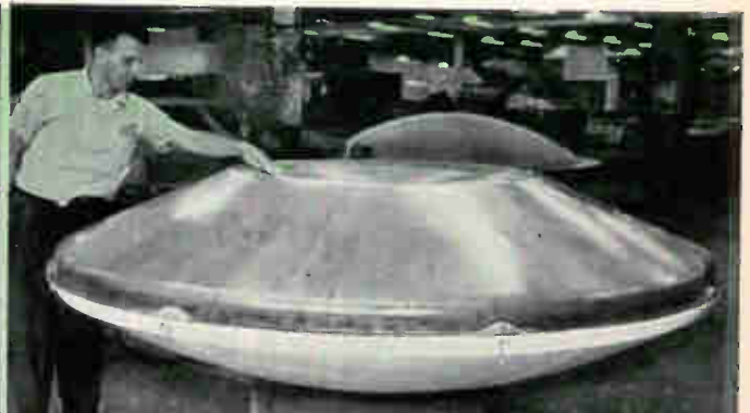
3 Cassegrain antenna built for U. S. Army Nike-Hercules radar
