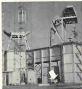
(Arrow points to truck. Compare Helix House size in first photo.) 8-story Helix House contains antenna coupling and automatic de-icing equipment to rid the immense antenna system of ice. Buried beneath the ground: another 11 million feet of copper wire in the radiating system terminating in the sea water itself.
