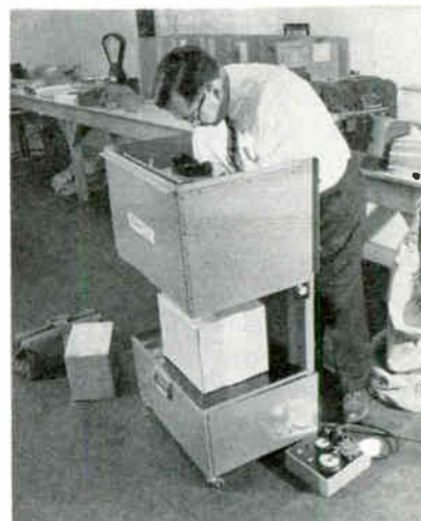
Portable x-ray unit (Westinghouse) weighs 160 lb, checks suspicious parcels of various dimensions
