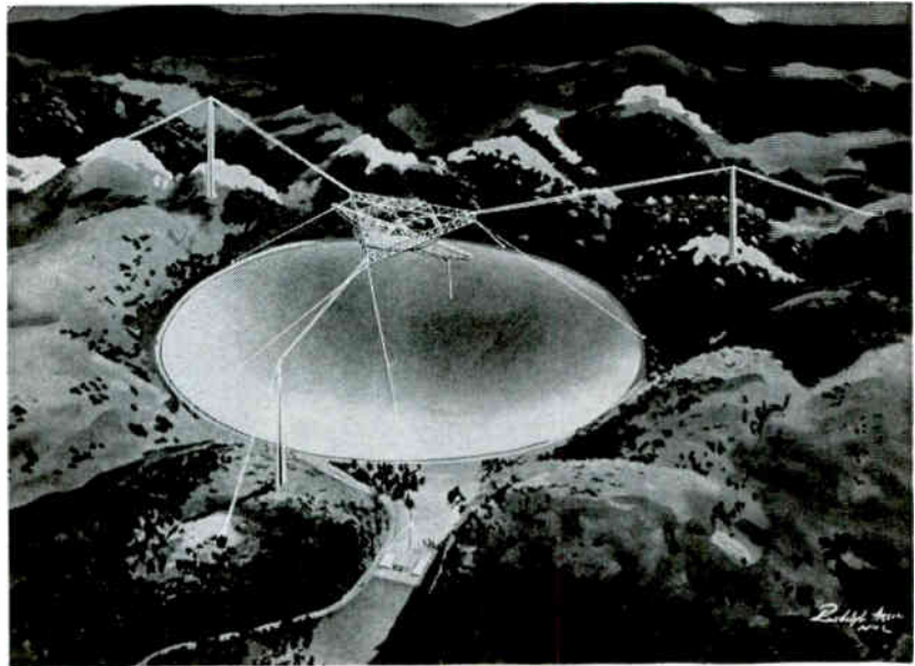
FIG. 1—Overall view of the Arecibo dish as it will appear when completed. Advantage is taken of natural dish-shaped valley
