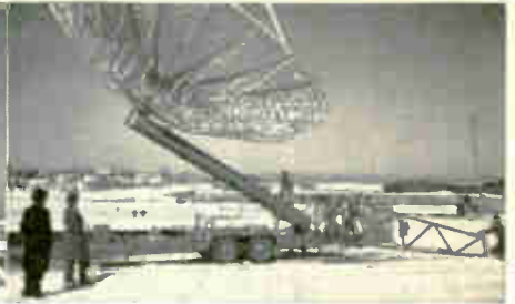
The antenna partially erected.
