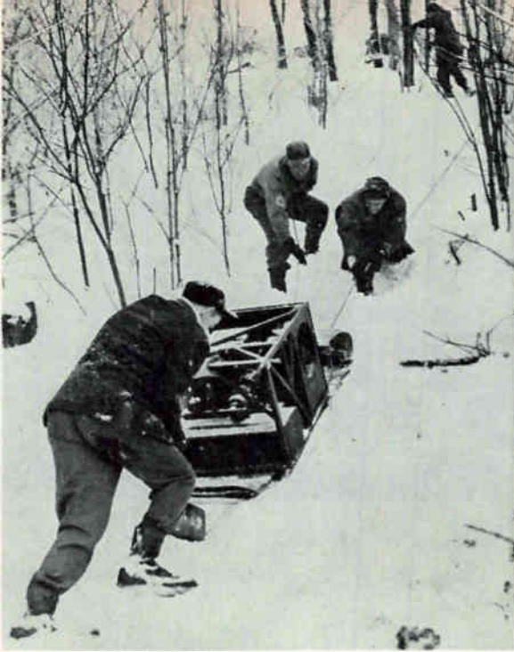
Sleds and muscles help field engineer bring equipment to snowy mountaintop military station
