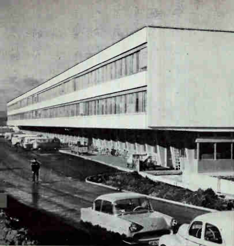
515 feet long, this cargo terminal office building at Zurich connects with warehouse, storage and cargo-handling building to the rear.
