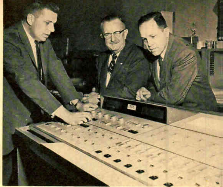
Engineers at Philadelphia Electric receive Honeywell computer-control system that assigns power generation requirements, provides cost data on grid interchanges
