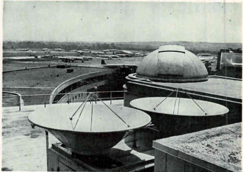
Use of separate transmitting and receiving antennas in K a band radar at Washington National Airport isolates crystal mixers from transmitted pulses by more than 95 db
