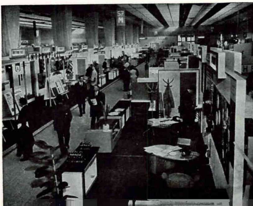
Booths at the Fourth International Electronics Components Show
